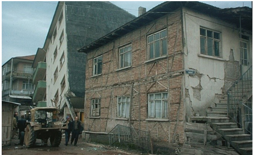
Structural failure in the concrete building in rear contrasts to the traditional building in front
